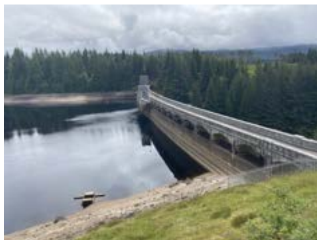
Laggan Dam on the River Spean in Lochaber, Scotland - part of the hydroelectric scheme that provides electricity to the Alvalde British Aluminium smelter in Fort William.
